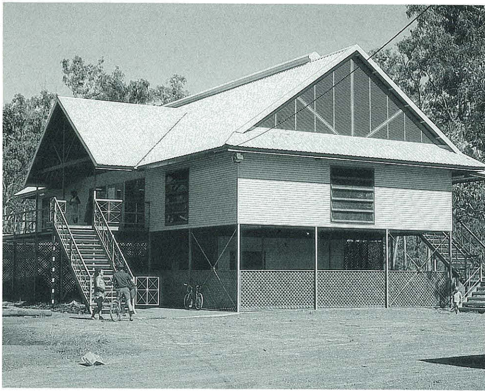
Community arts building at Ramangining, Arnhem Land. Photo: Karen Coote.
